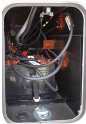
Typical Class A motorhome auxiliary battery compartment
