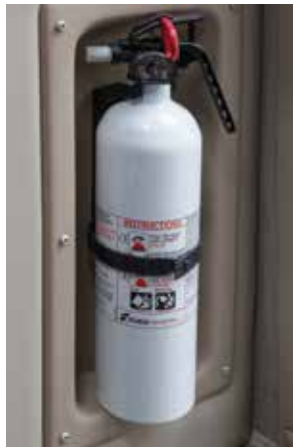
Typical Class B-C fire extinguisher
